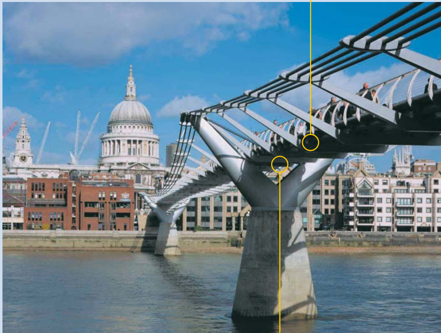
Millenium Bridge – London, GB
