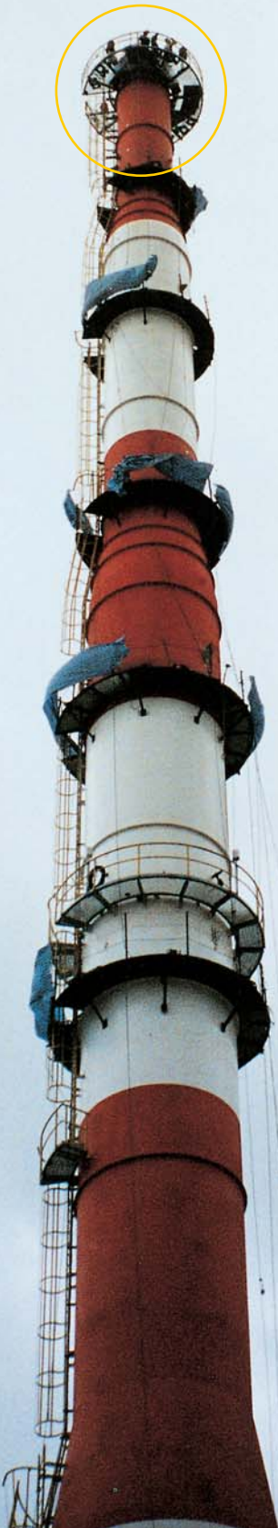
Chimney – Thailand (Ringdamper)
